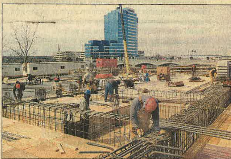
Workers place steel reinforcement rods.
