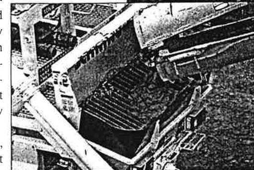
Left: Concrete is loaded into a Schwing pump.
